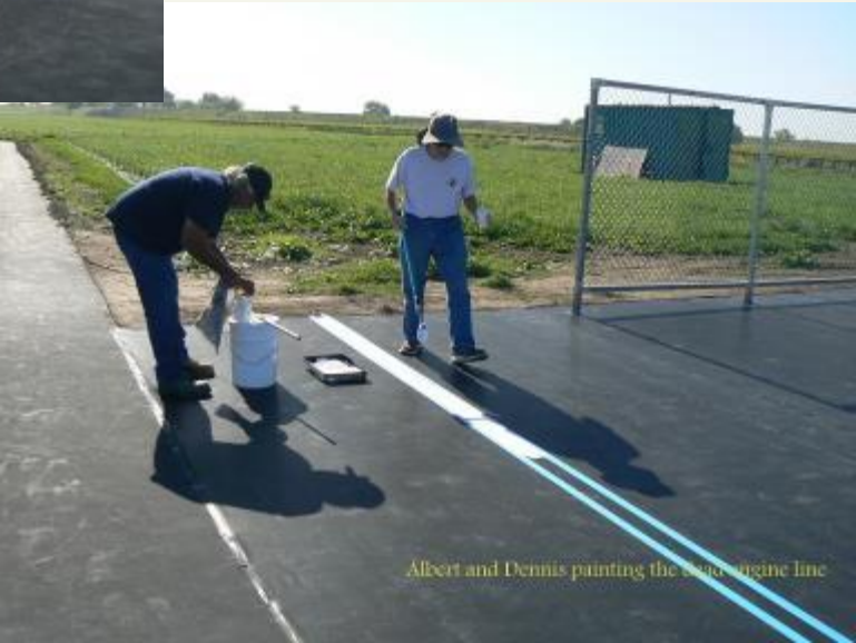
Roofing going on the shade structure
